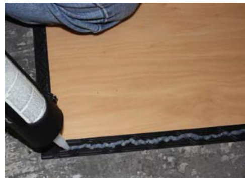
Seam sealer for waterproof installation
